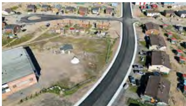
Top Photo: Pool and Youth Centre Being Built in Whapmagoostui
