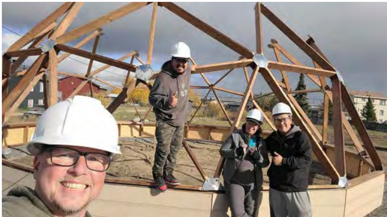
CERRI Geodesic Dome, Chisasibi
