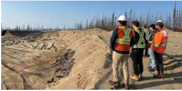
Visit of the new landfill being built in Whapmagoostui
