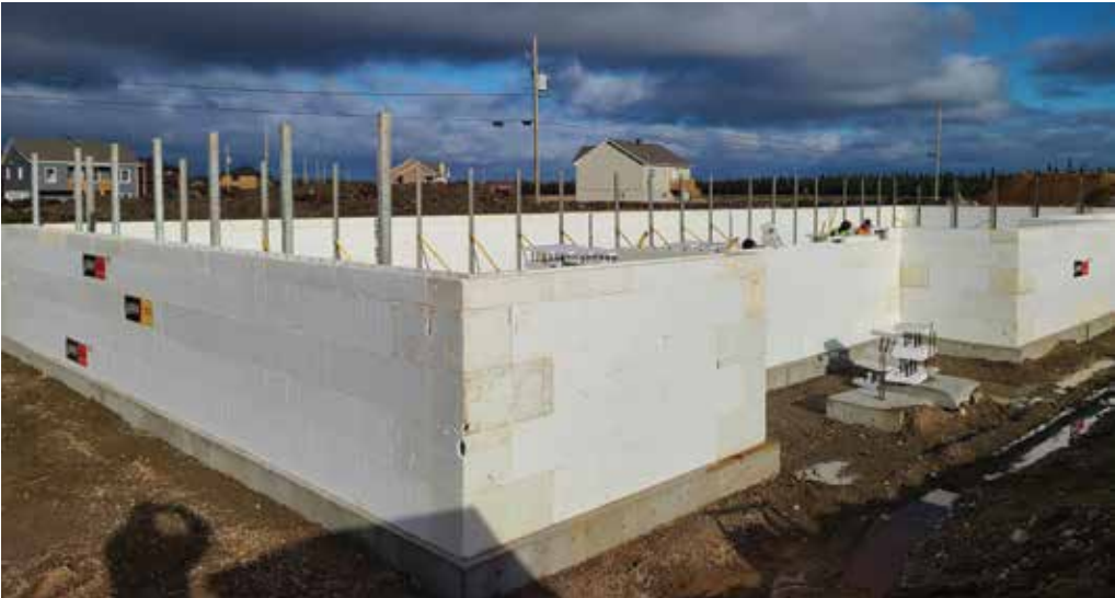
Modular units' foundation
