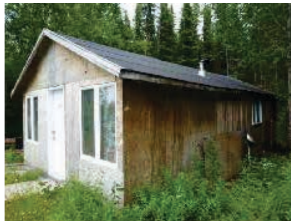
Cabin renovation (2016 Enhancement project) visited July 2017 (Clarence Blacksmith, Land User; Frank Blacksmith, Tally Person)
