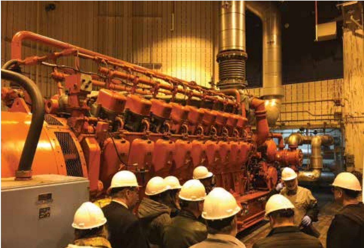
Tour of the Jean R. Marcotte Wastewater Treatment Plant November 15, 2017
